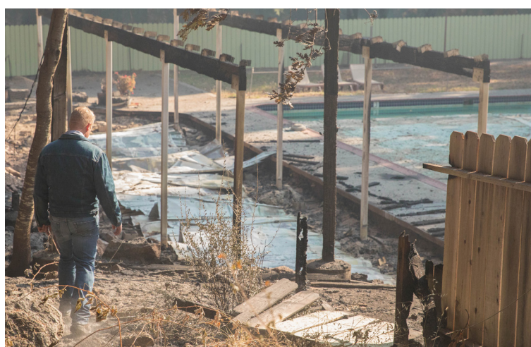
Photos from top to bottom: 1. The burnt out staff house. 2. The pool and demolished pool house at Enchanted Hills Camp. Opposite: >> EHC Staff and youth camper work on paper mache together.
